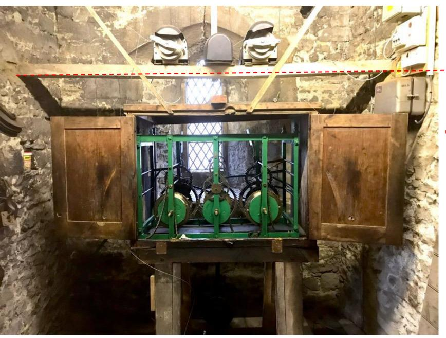
Line clearly shows the bowed support beam. This needs to be replated with a larger hardwood alternative.
